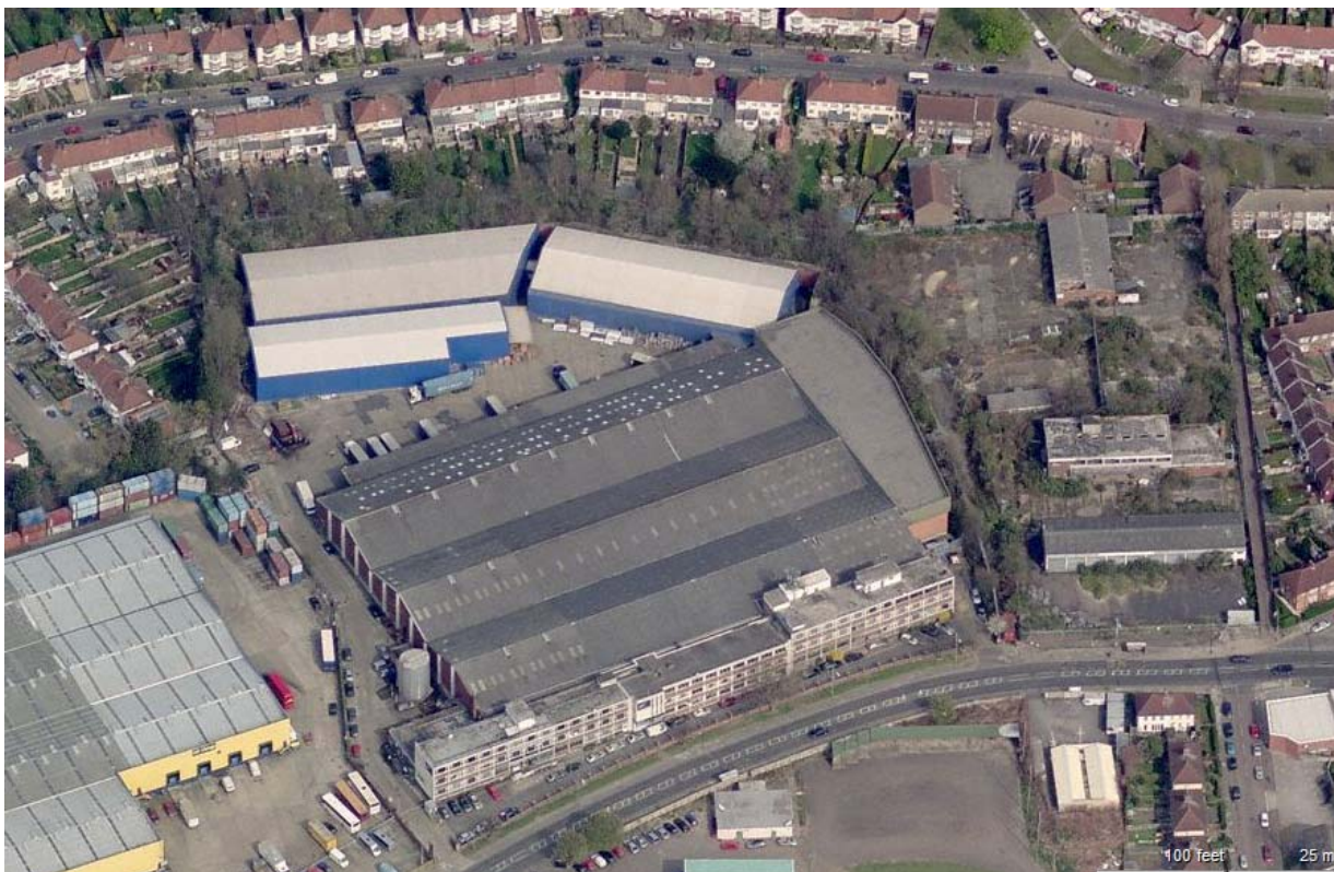
Figure 1: Aerial Photo of Previous Site Layout
